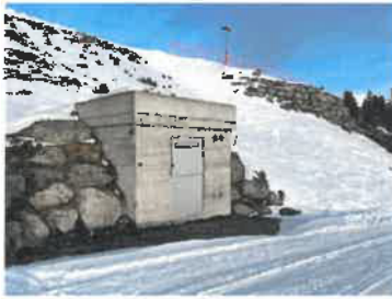
Alpine Photovoltaik-Grossanlagen in Klosters Züg Klosters
